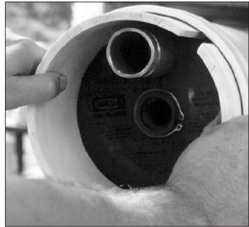
Fig. 2.1.16 - Installing head using insertion tool
