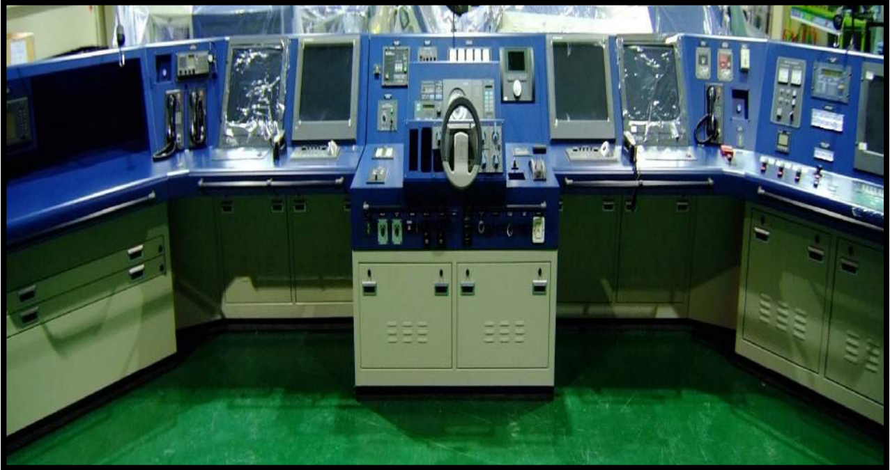
[Bridge Control Panel]
